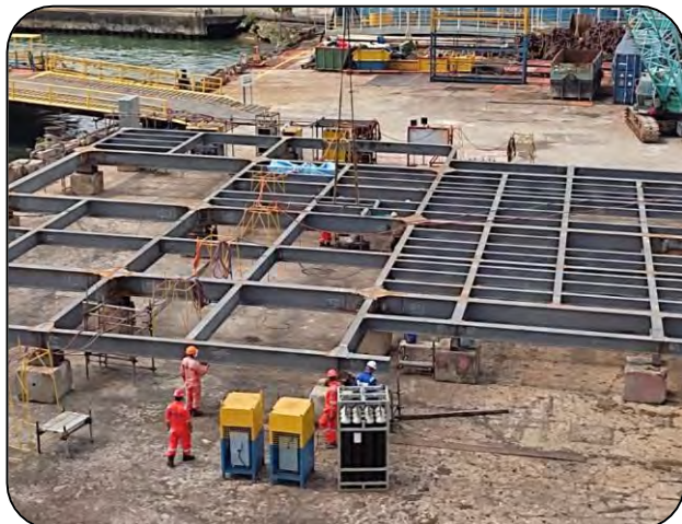
Assembly of super structure at open yard
