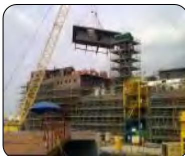
Accommodation Erection
