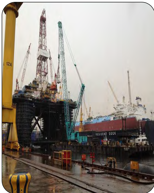
Kim Heng 55 Crane Barge Lifting of LMRP & BOP Assembly from Rig
