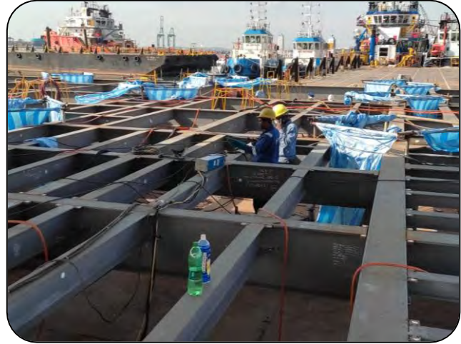
Fabrication of superstructure in segments
