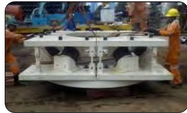
Setting of Gimbal on Load Plate
