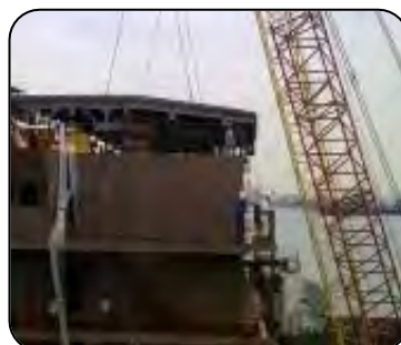
Heli-Deck Erection
