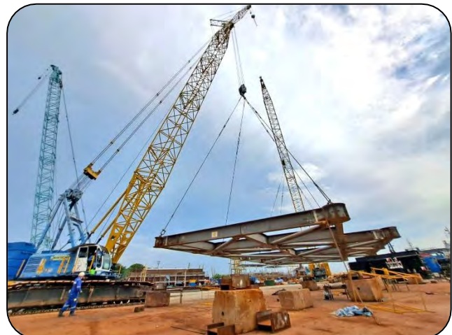
Assembly of super structure at open yard
