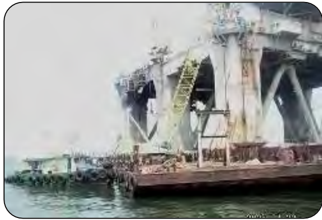
Mobilization of Crane Barge and equipment alongside.
