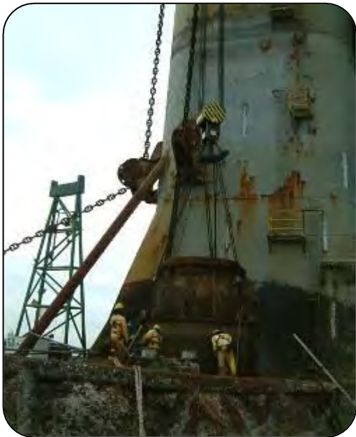
Lifting of Thruster Unit
