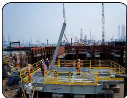
Tension Deck Arm Installation and Trial Function Test
