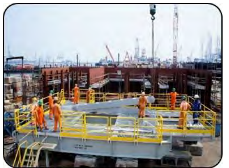
Tension Deck Arm Installation and Trial Function Test
