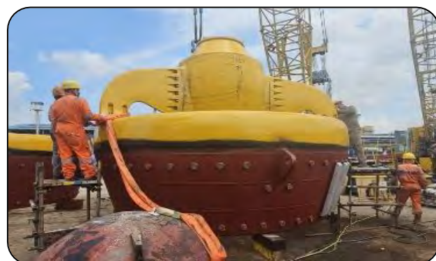
Main thruster assembly at open yard
