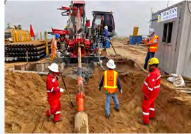
Horizontal Directional Drilling (HDD)
