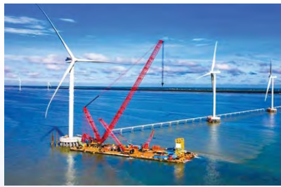
Crane Lifting Solutions
